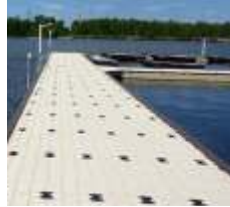
PUBLIC PIERS, DOCKS
